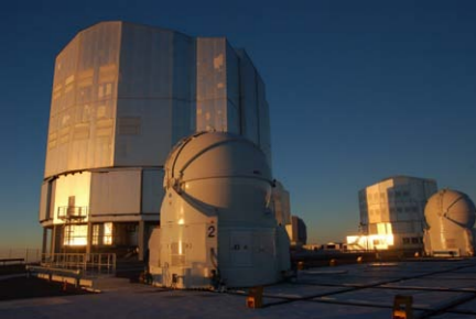
Figure 1: Astronomical Interferometers such as the Very Large Telescope Interferometer (VLTi) at Cerro Paranal in Chile deliver images with the resolution of a telescope of 100 meter diameter, by means of a few smaller telescope (diameters: 1.8 m or 8 m).
